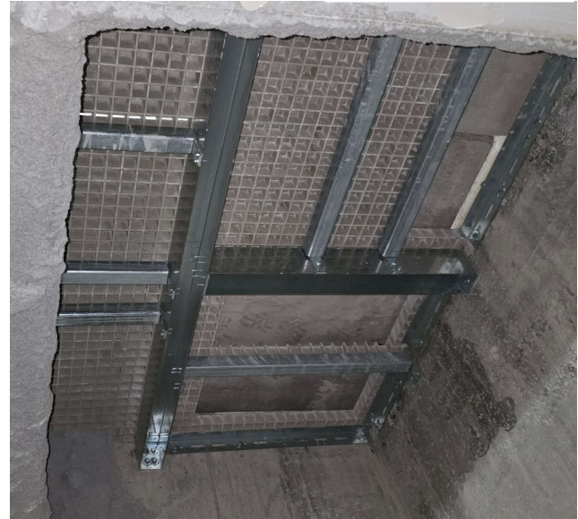
Retrofit access flooring in service riser void
