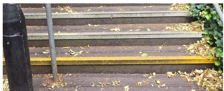
Recycled plastic footpath planks and GRP nosings
