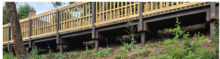
Recycled plastic structural posts, beams and joists
