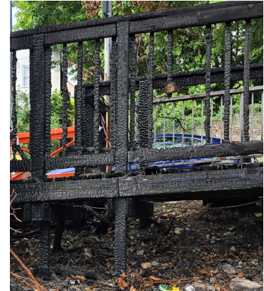
Original rotten and fire-damaged timber walkway
