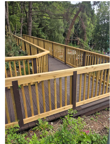
Recycled plastic structural posts, beams and joists
