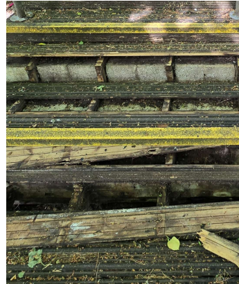
Original rotten and fire-damaged timber walkway
